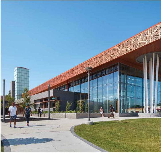
ROUTE 9 LIBRARY AND INNOVATION CENTER New Castle, DE
