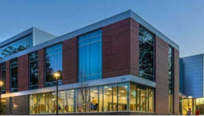
Foundation YMCA Wilson, NC Little
