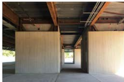
Ground Level Before Renovation
