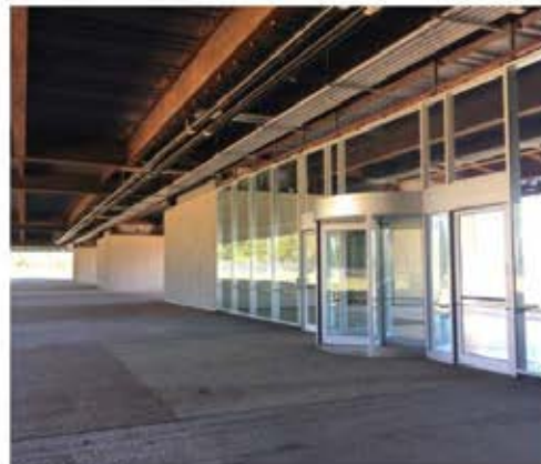
Main Entry Before Renovation
