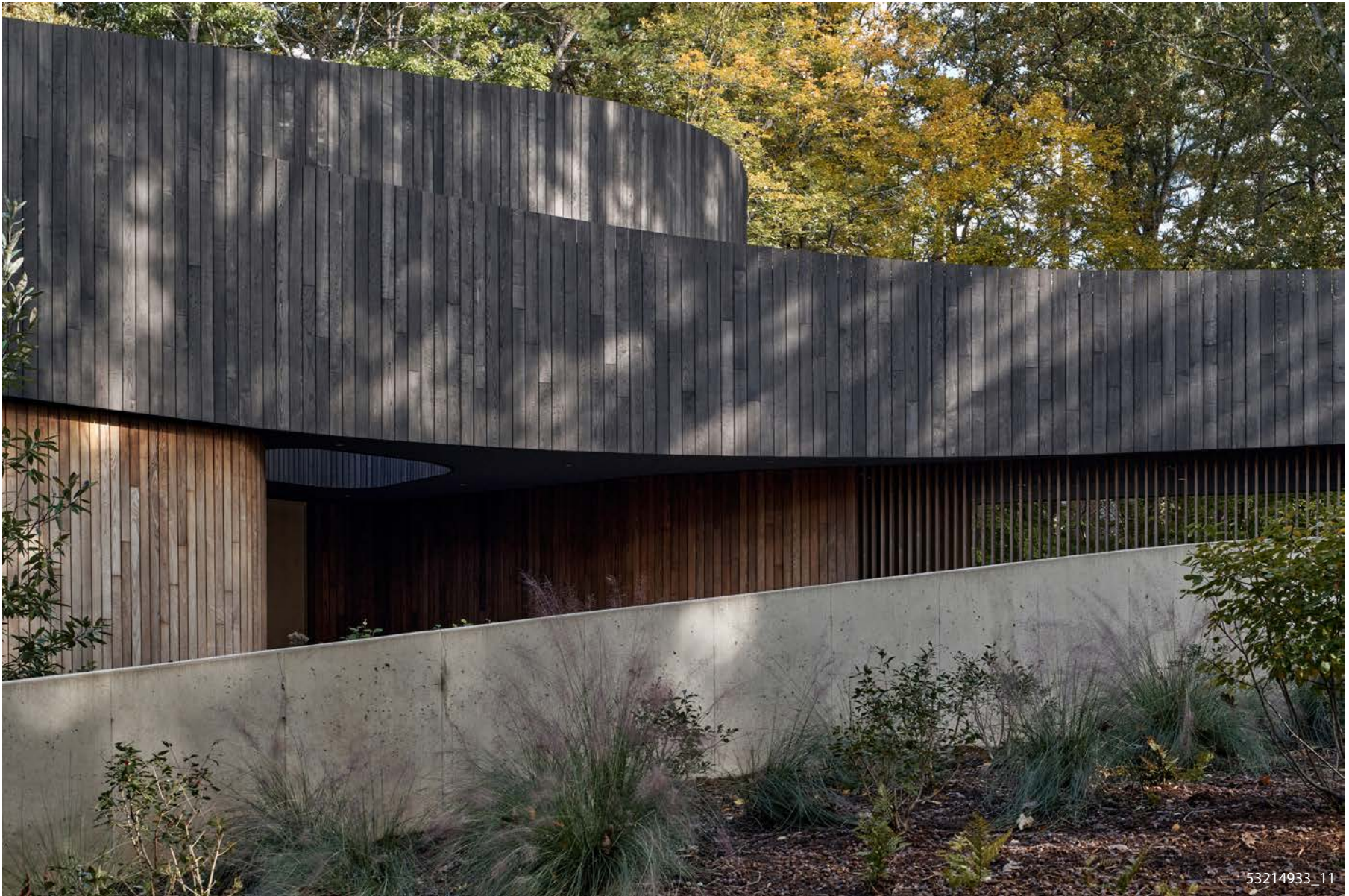
The front of the house is solid, an interwoven landscape of site walls, reentrant ground level folds, and sweeping forms above that greets the neighborhood as a sculptural volume.
