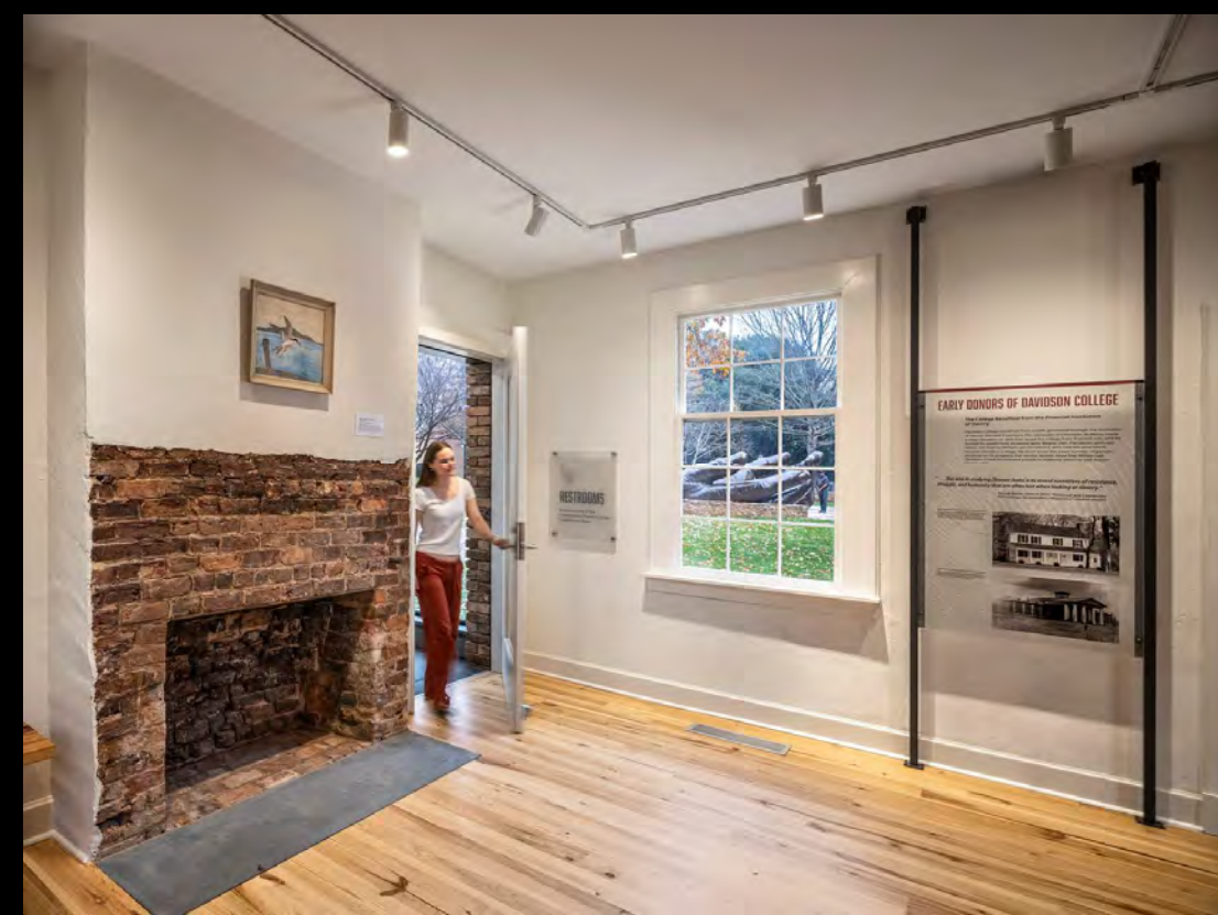
Reclaimed bricks from demolition were used to repair and stabilize the new openings and uncovered original fireboxes.
