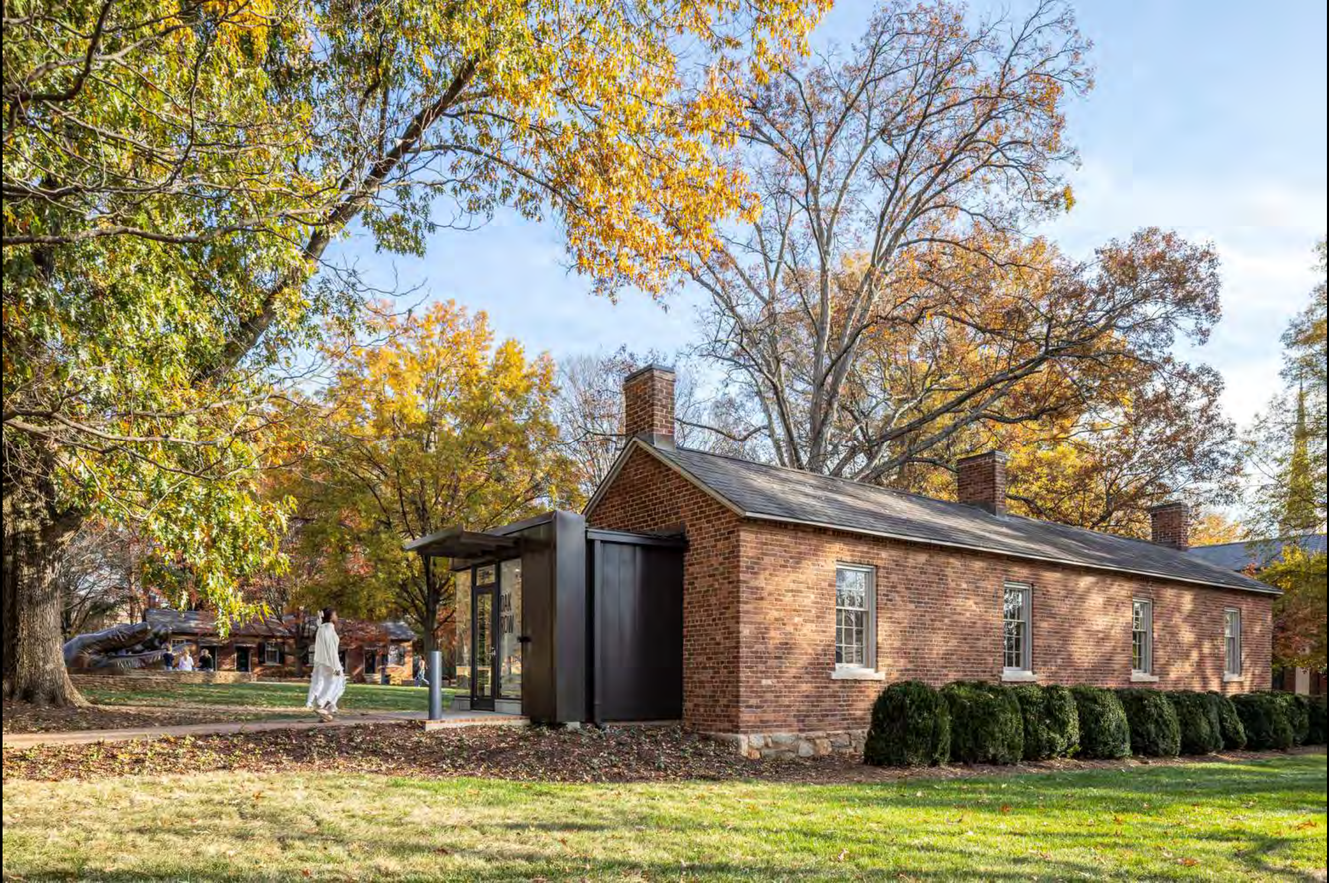
View from the northwest corner of the site shows new vestibule and sculpture beyond.
