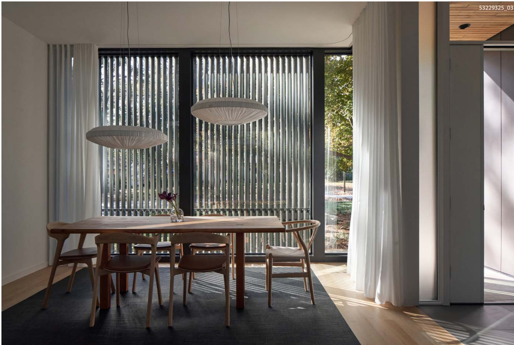
A movable slat wall over the front window allows the clients to close the house when they are away for long periods of time.
