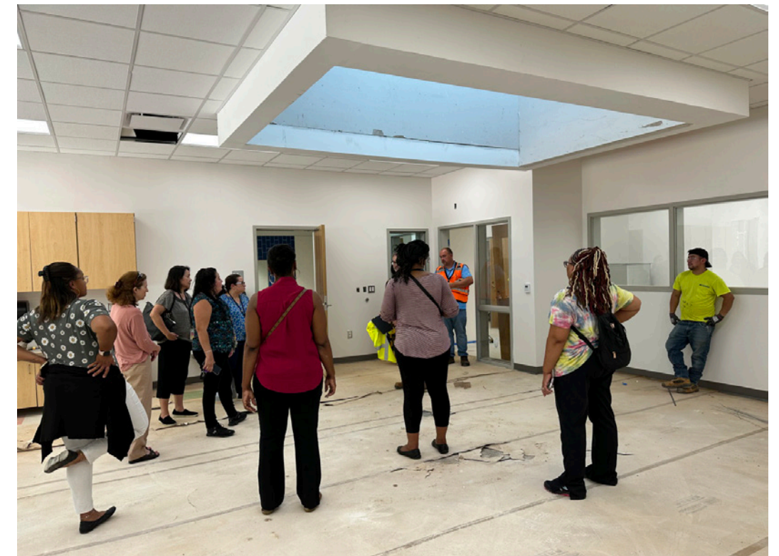
School leaders and educators tour the classrooms with building contractors present to observe and plan for their new teaching environments
